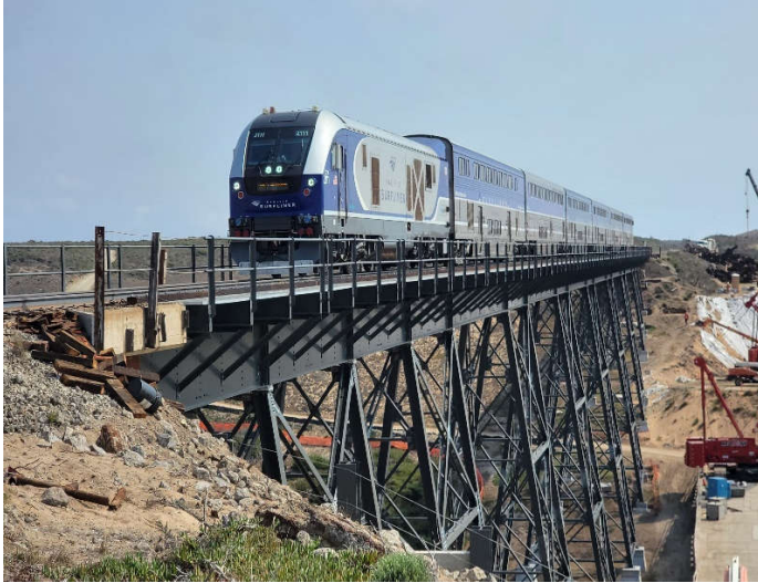
Narlon Bridge Replacement, Source: UPRR
