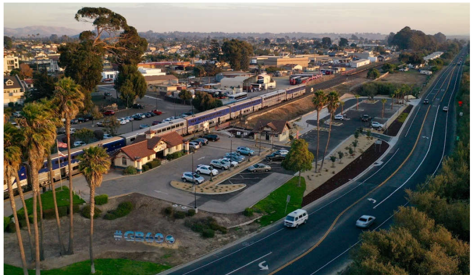
Grover Beach Station Expansion, Source: City of Grover Beach
