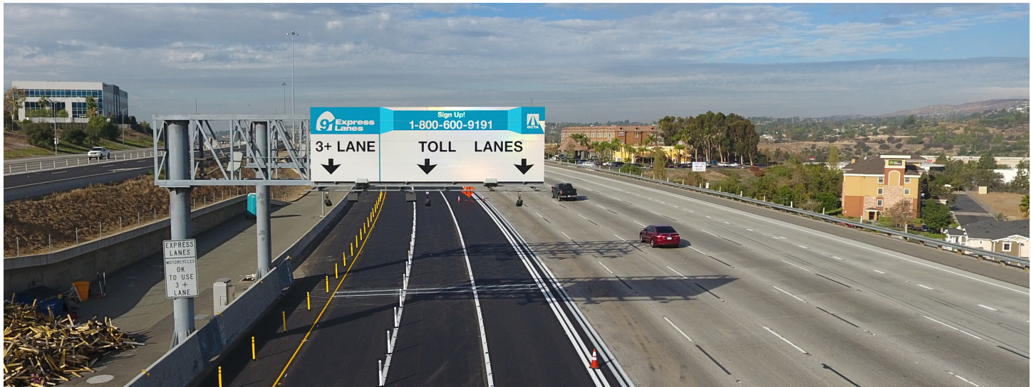
The Pavement Replacement Project on the 91 Express Lanes was completed in 2016.
