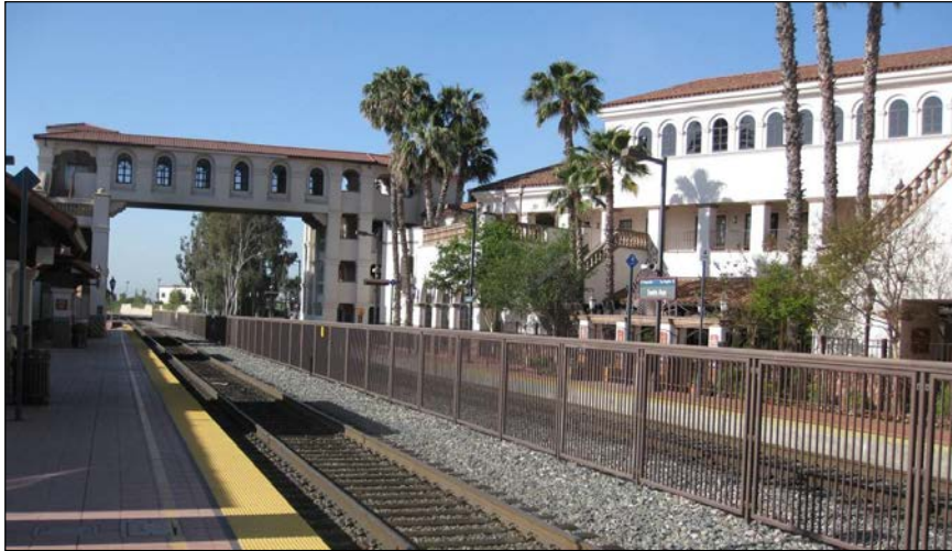
Station platform and pedestrian overcrossing.
