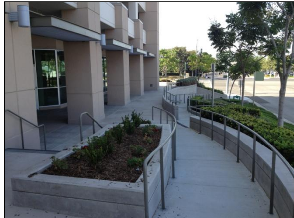
Pedestrian ramps leading to Barranca Parkway.
