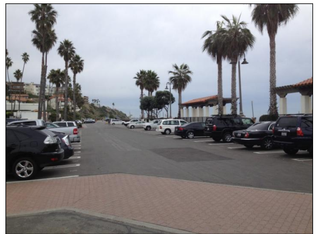
Parking lot with crosswalk pavers.
