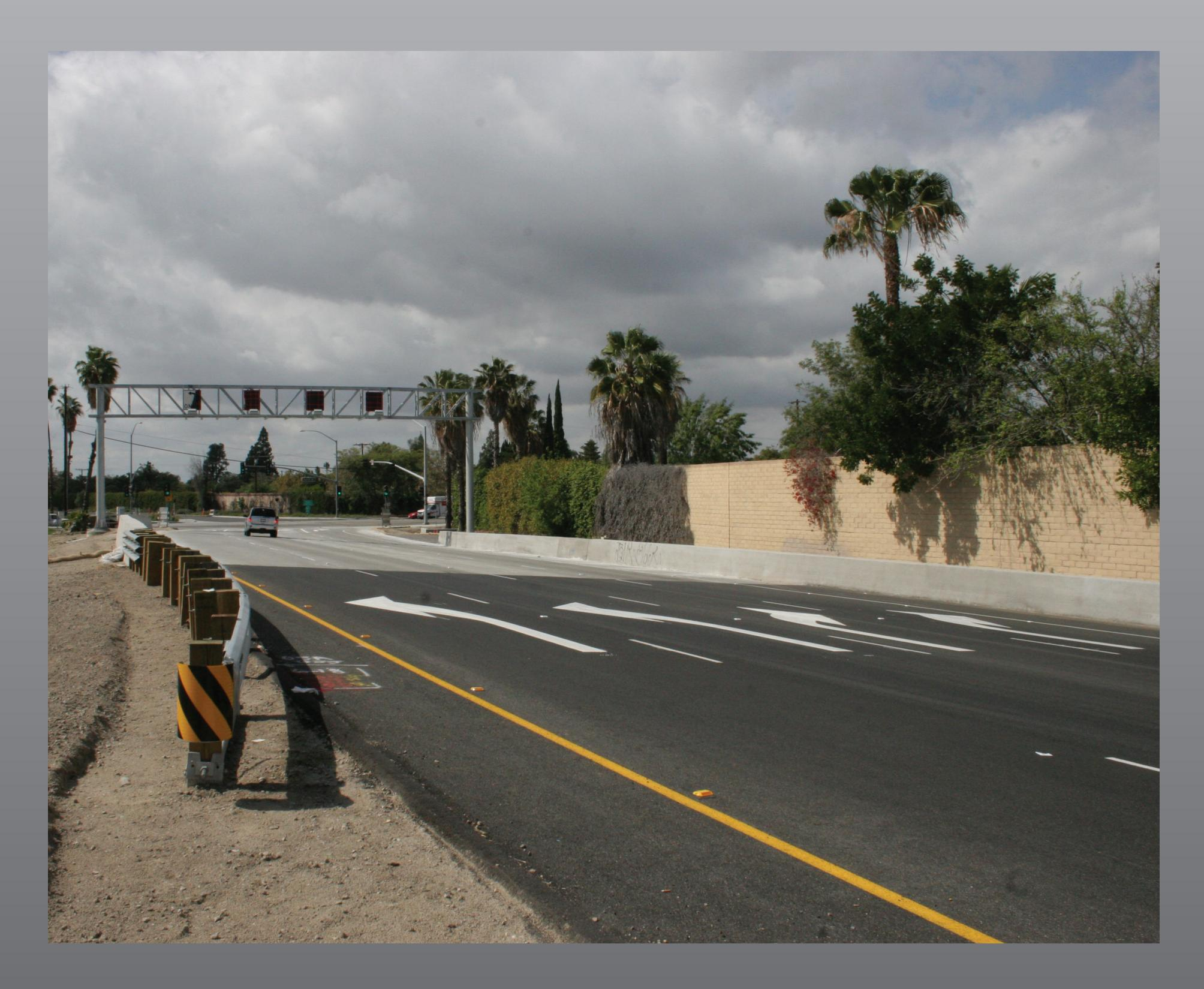
Ten westbound on- and off-ramps were realigned and reconstructed to create a smoother and safer transition for motorists. The improved ramps also provide dual exit lanes, added capacity and dedicated turn lanes to reduce back-up on the freeway and to streamline transition from the freeway to local streets.
