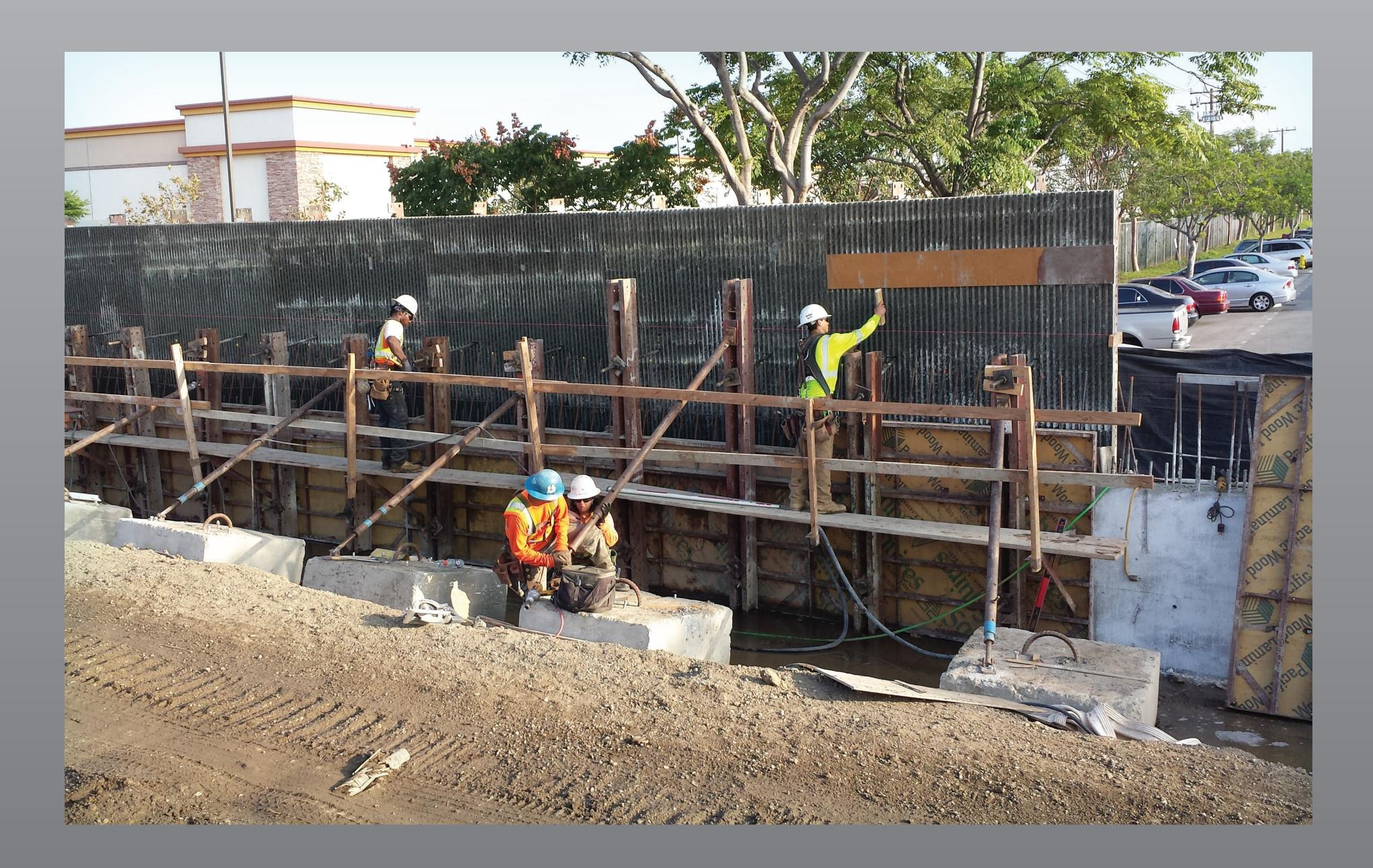
Twelve retaining and/or sound walls were constructed along the project corridor to reduce erosion, provide structural support and deliver noise mitigation. Throughout the project, more than 1.9 million pounds of steel and 35,000 square feet of masonry block were incorporated.
