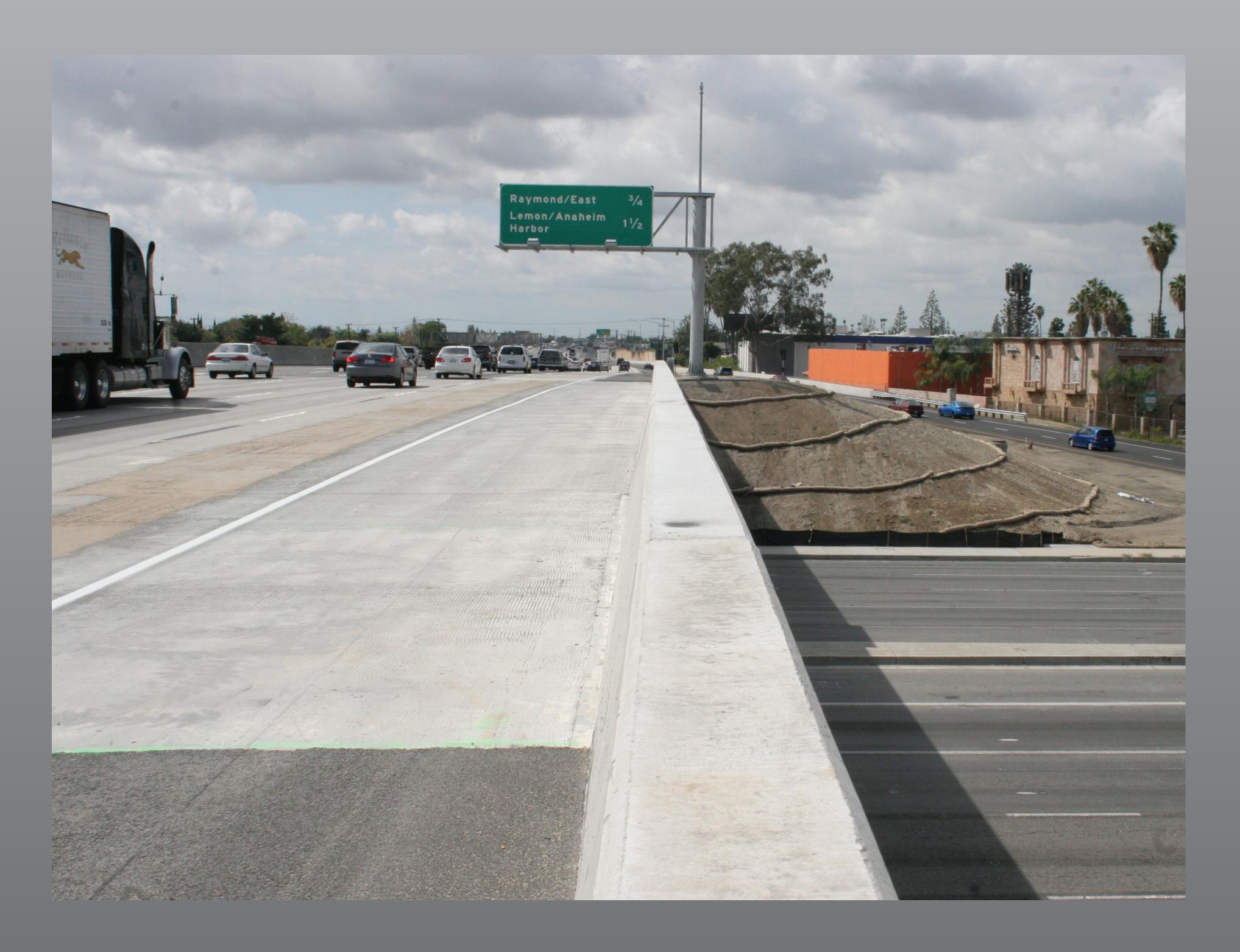
In addition to the new lane, auxiliary lanes were constructed between most exits to ease merging operations, reduce chokepoints and enhance safety. New striping, overhead signage and barriers were implemented throughout the project corridor to provide enhanced visibility and safety for motorists.
