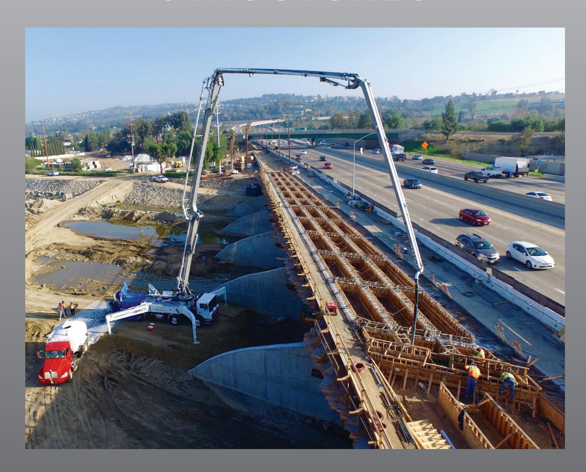
To make way for the new lane, the Santa Ana River Bridge was widened and nine retaining walls were reconstructed along westbound SR-91. To deliver these structural improvements, 17 piers were extended, 16,000 linear feet of piles were driven and 13,500 linear feet of soil nail were incorporated.
