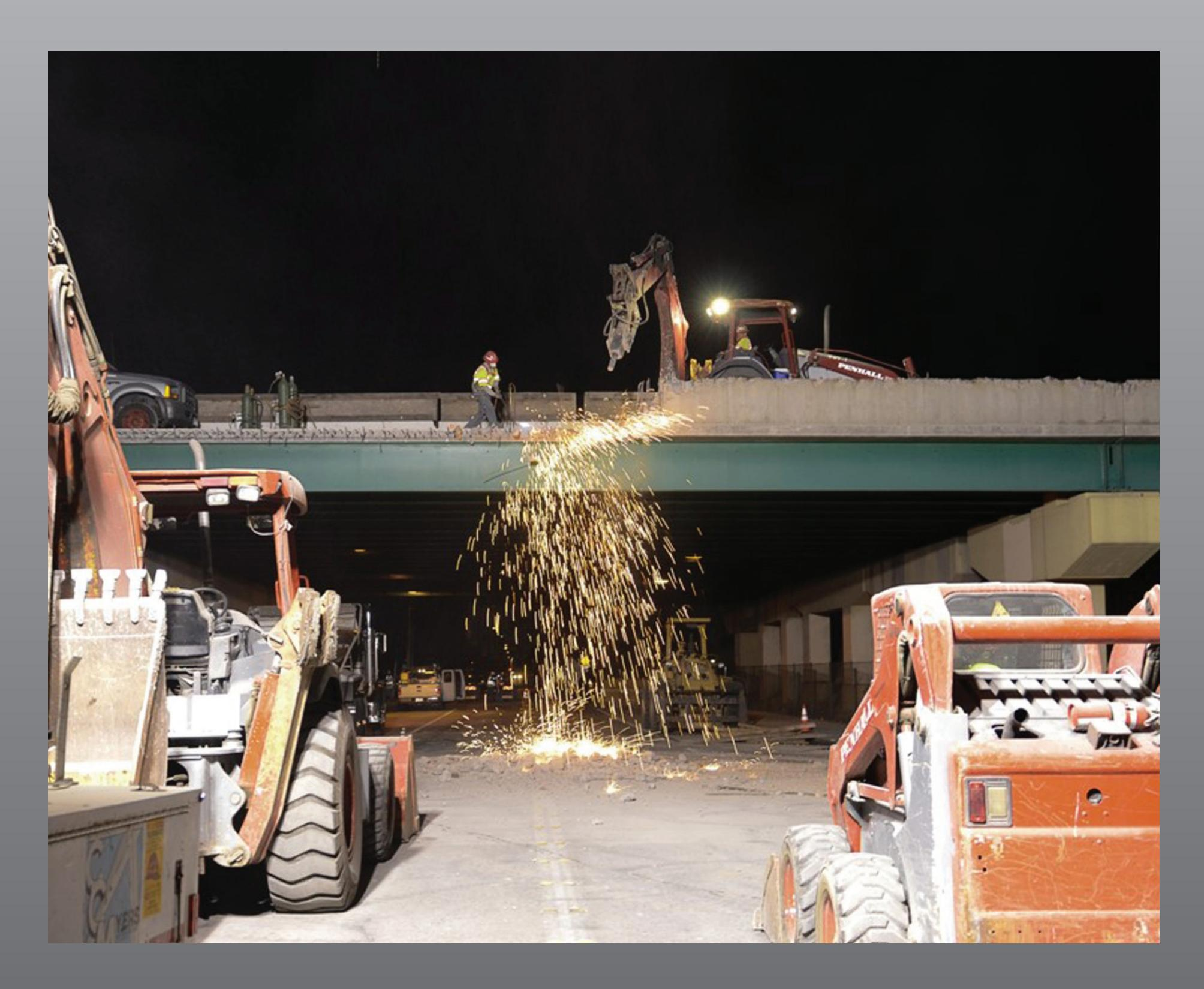
As part of the SR-91 Westbound Lane Addition Project, construction crews widened six bridges in the westbound direction. The widened overcrossings cleared the way for the new lane, standardized lane and ramp widths, dual exit lanes at ramps, and facilitated incorporation of underground drainage systems and new safety features.
