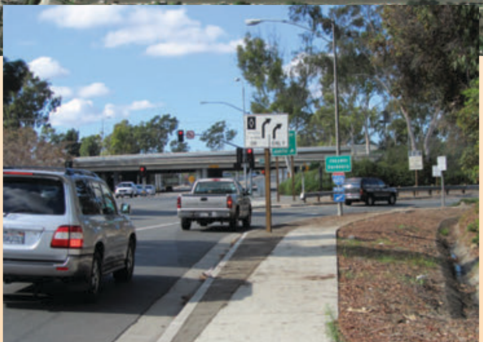
Enhancing Safety Northbound ramp onto I-605
