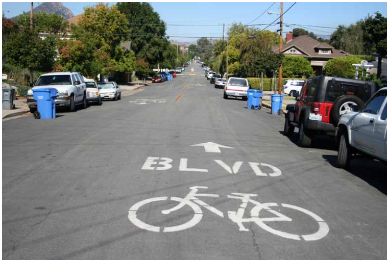
Bicycle Boulevard pavement symbols (San Luis Obispo, CA) Photo credit: Mike Singleton
