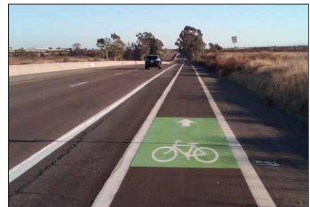
Buffered bike lane on Kearny Villa Road. (San Diego, CA) Photo credit: Joe Punsalan
