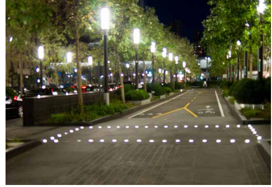
Example of in-pavement flashing crosswalks Photo Credit: bicyclinginfo.org
