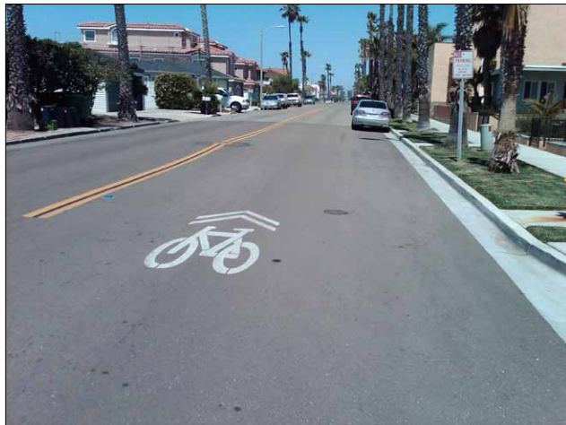
Shared Lane Marking (Oceanside, CA) Photo credit: John Holloway
