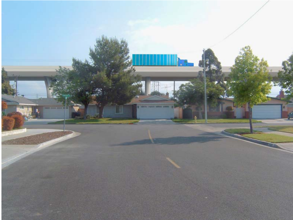
Figure 5-2 Viaduct Renderings – Upper: Viaduct at Two Levels above Grade to Clear a Nearby Arterial Over Crossing of the Freeway as seen from Laura Way in Westminster – Lower: Viaduct at a Single Level above Grade as seen from Duncannon Avenue in Westminster
