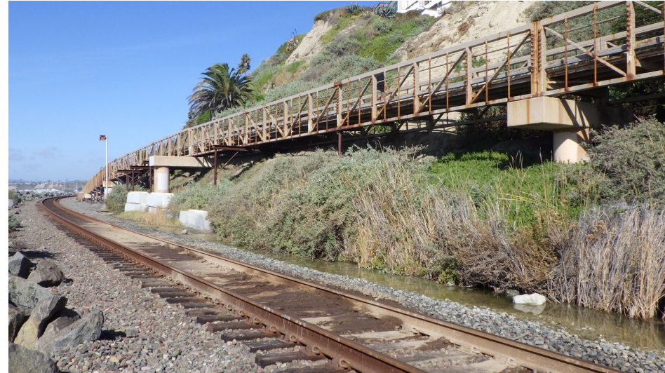
Monitoring Areas #4, 5 MP 204.00 – 204.30 Mariposa Pedestrian Bridge, MP 204.50 – Linda Lane
