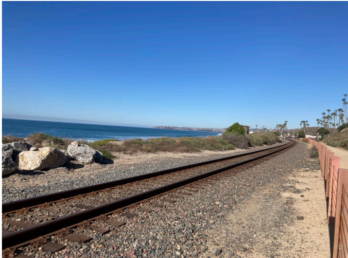
Monitoring Area #3 MP 203.65 - 203.70 North Beach
